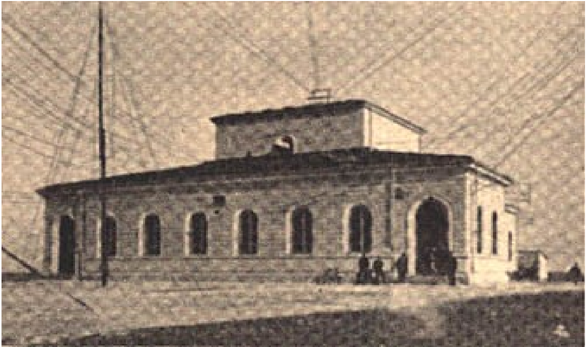
Another perspective of the headquarters of the Palazzina Marconi Radio Station
